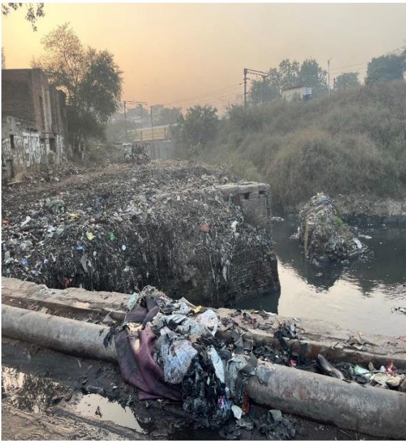
Fig. 7 Location: Open drain near Agra Fort Station
